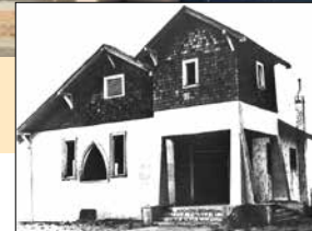
First Baptist Church (restored)
