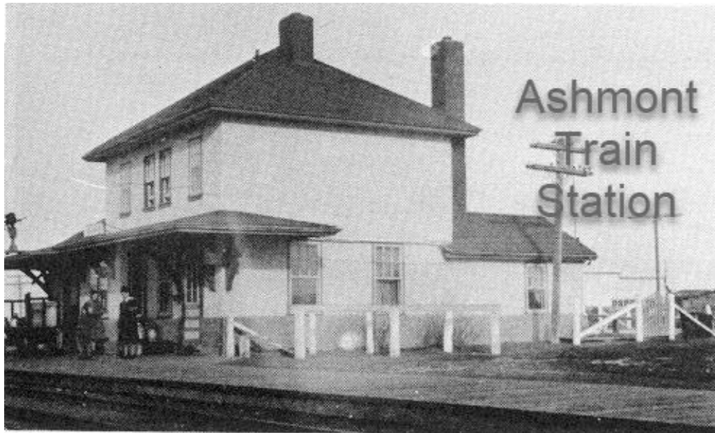
Ashmont Station House 1942
