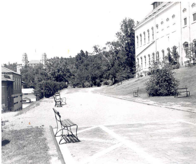
Completed brickwork on south promenade.
