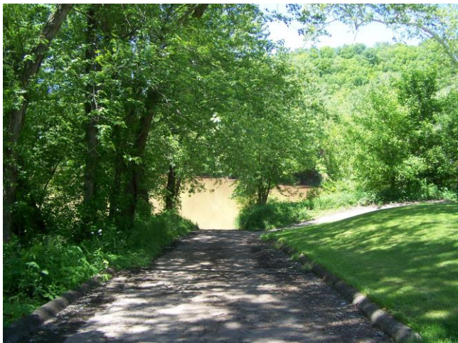
Spring Valley-Mouth of Hughes (Map Tag 35), a single lane concrete ramp.
