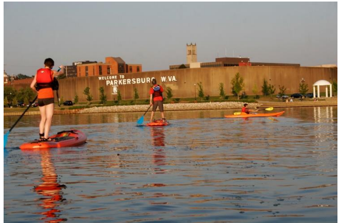
Parkersburg Flood Wall, Ohio River. Photo John Wiseman
